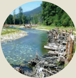
Large Wood Installation
