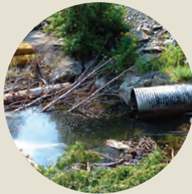
Culvert Renovation & Fish Passage Barriers
