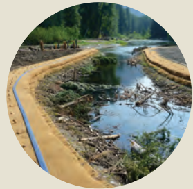
Floodplain & Side Channel Reconnection
